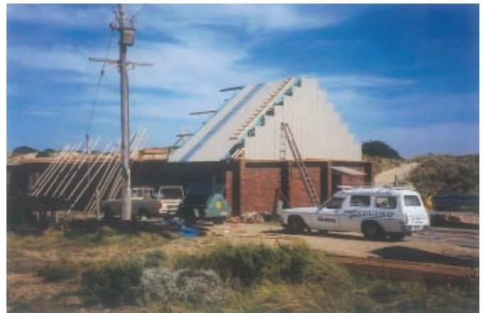
This was an exciting and rewarding experience for all those involved. Under the guidance of two tradesmen, members of the Club removed the old roof, erected trusses and clad the roof. All work was completed in time to start the new patrol season.
